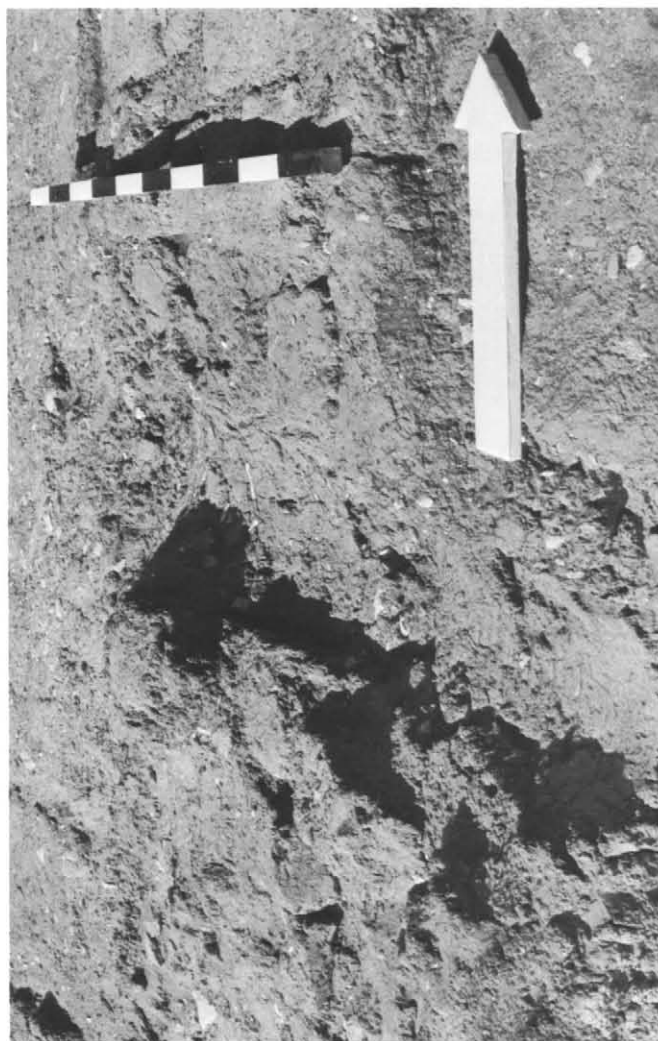
Pl. 10d: Drain channel through brick causeway wall.
