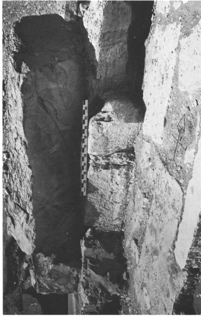
Pl. 19d: Core masonry of the room of the five niches from the east.
