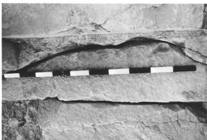
Pl. 41a: Socket for patching slab over ancient cracks in the casing of the north side of the pyramid.
