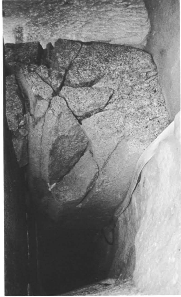
Pl. 44c: Crushed lower end of second plug in entrance corridor. See pl. 89.
