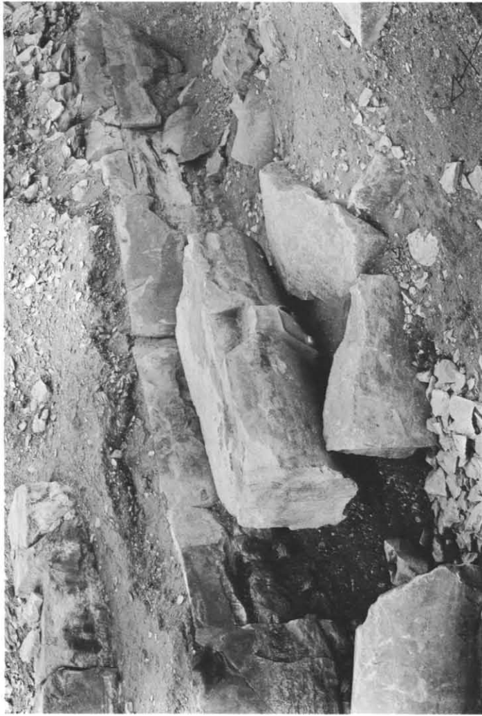
Pl. 28b: South wall of inner enclosures with coping block. See fig. 21.
