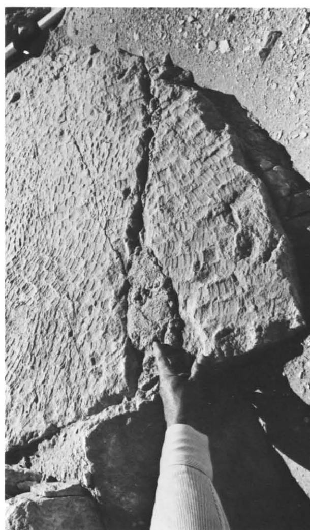
Pl. 41c: Mortar used to repair crack in casing block.
