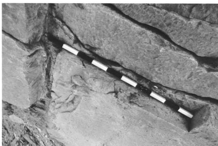
Pl. 41a: Socket for patching slab over ancient cracks in the casing of the north side of the pyramid.
