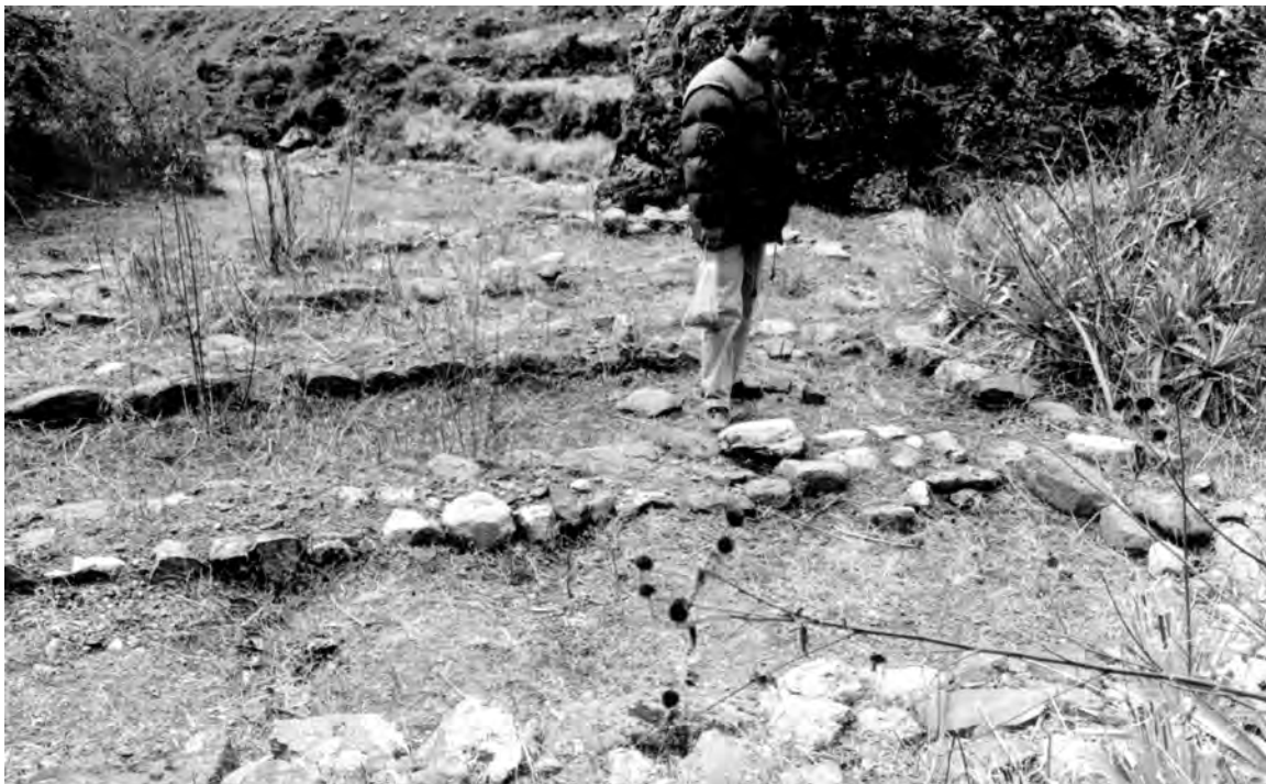
FIGURE 15.23. Foundation of storage-structure-like building, lower-altitude site
