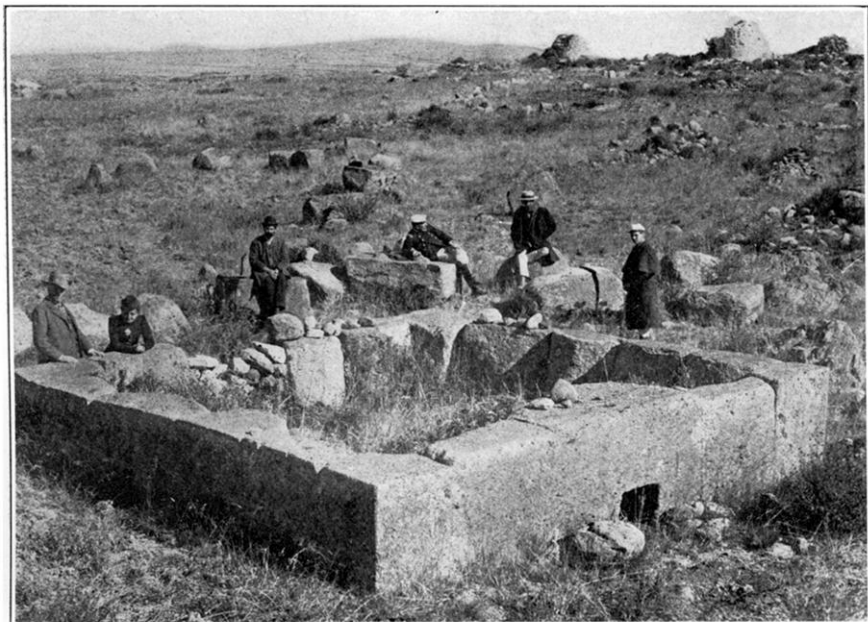
1. Quadrangular Structure k .
