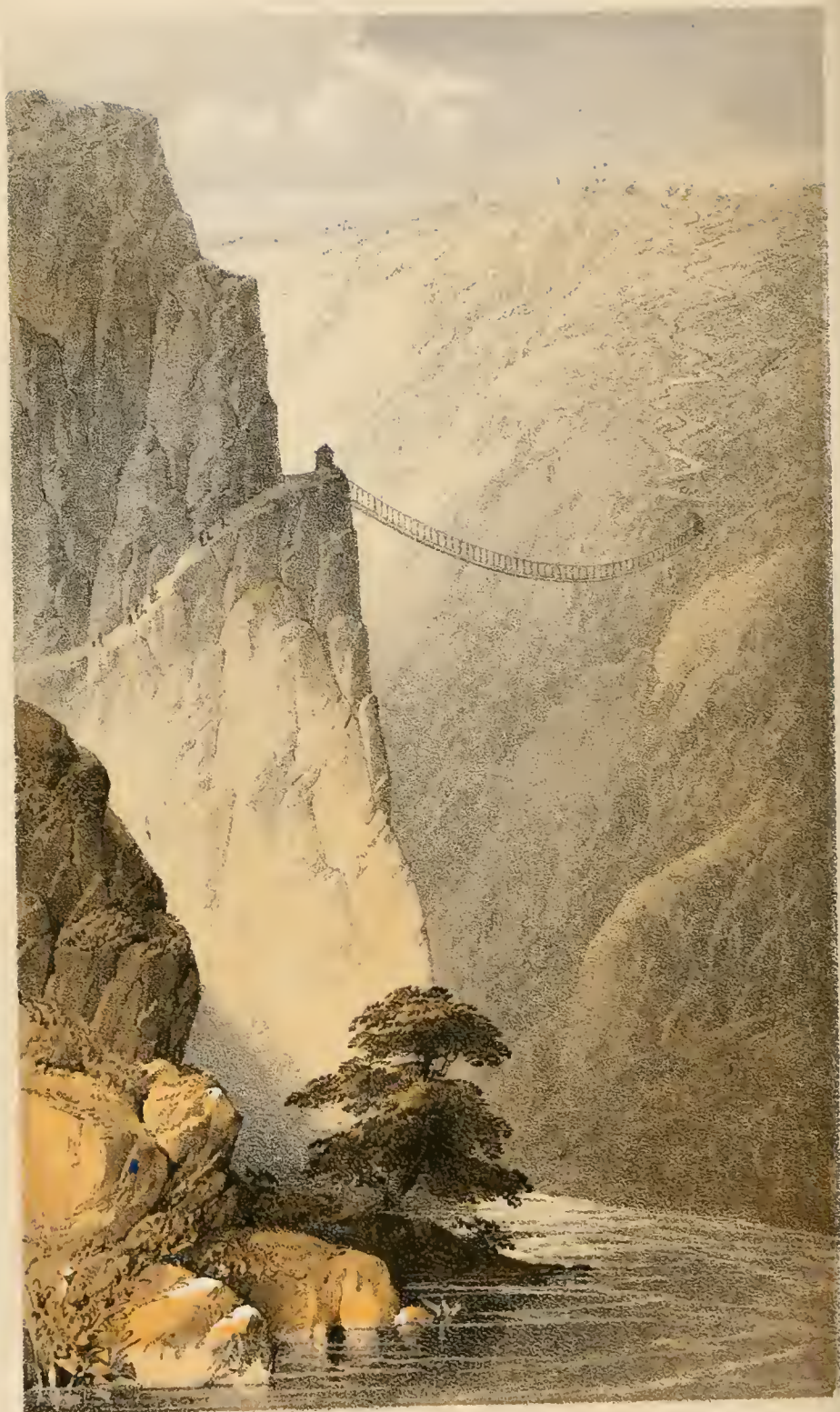
THE SUSPENSION BRIDGE
