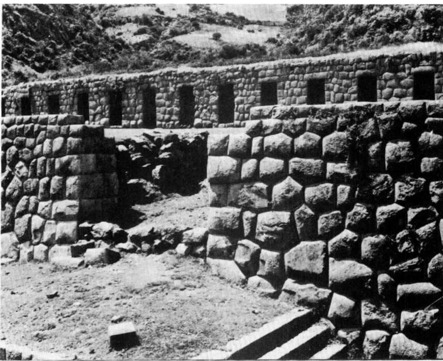
15 Polygonal Inca masonry in the terraces of Tarahuasi, Limatambo, below the hill of Vilcaconga
