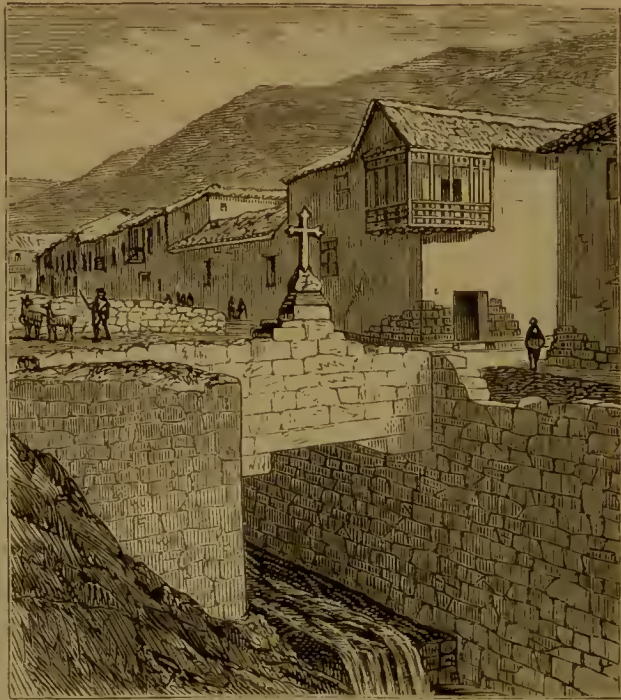
INCA BRIDGE OVER THE HUATENAY, CUZCO.
