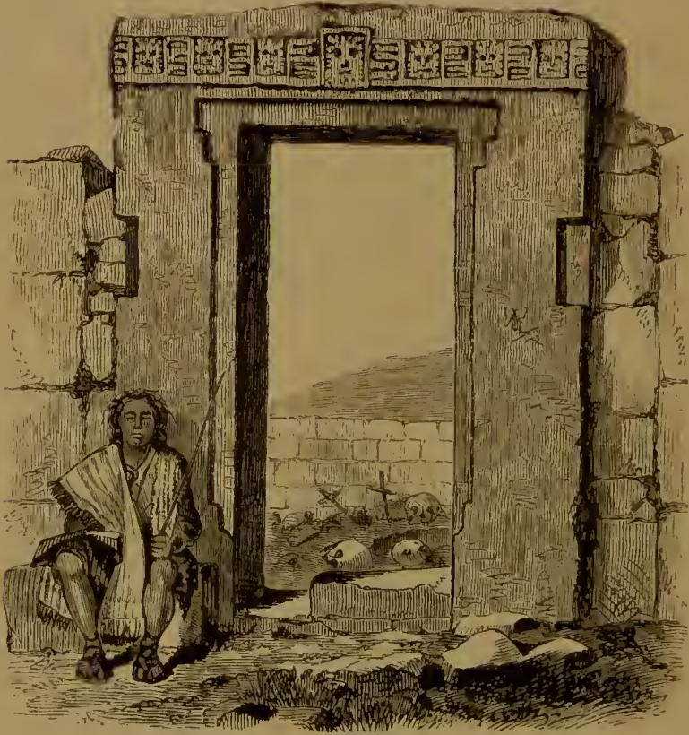
GATE-WAY AT CEMETERY—FRONT VIEW.
