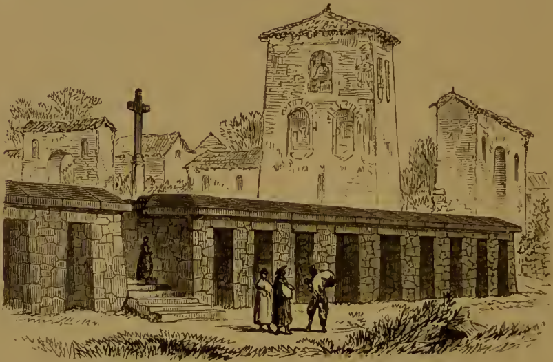
COPED AND NICHED TERRACE WALLS, CHINCHERO.
