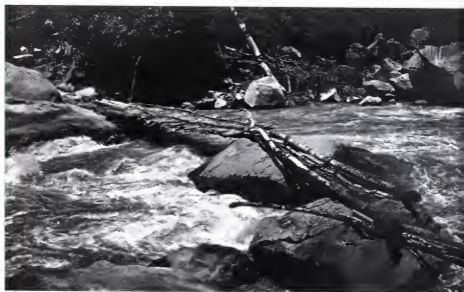
'Heald's Bridge across the Urubamba, 1912.'
