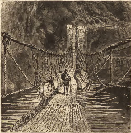
LOOKING ACROSS THE BRIDGE.
