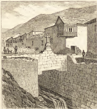
INCA BRIDGE OVER THE HUATENAY, CUZCO.
