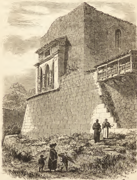
END WALL OF THE TEMPLE OF THE SUN, CUZCO.
