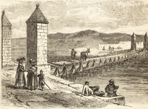
BALSA BRIDGE OVER THE RIO DESAGUADERO.
