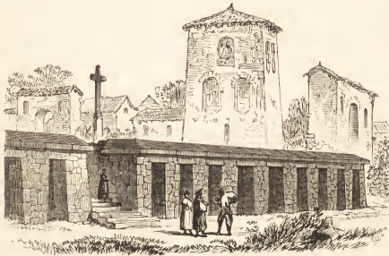
COPED AND NICHED TERRACE WALLS, CHINCHERO.
