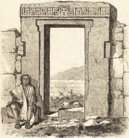
GATE-WAY AT CEMETERY—FRONT VIEW.
